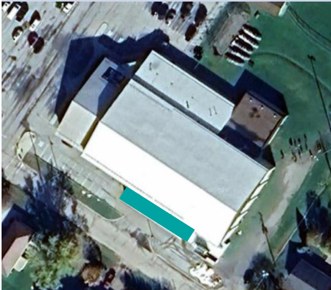
Hagersville Arena: Aerial View
