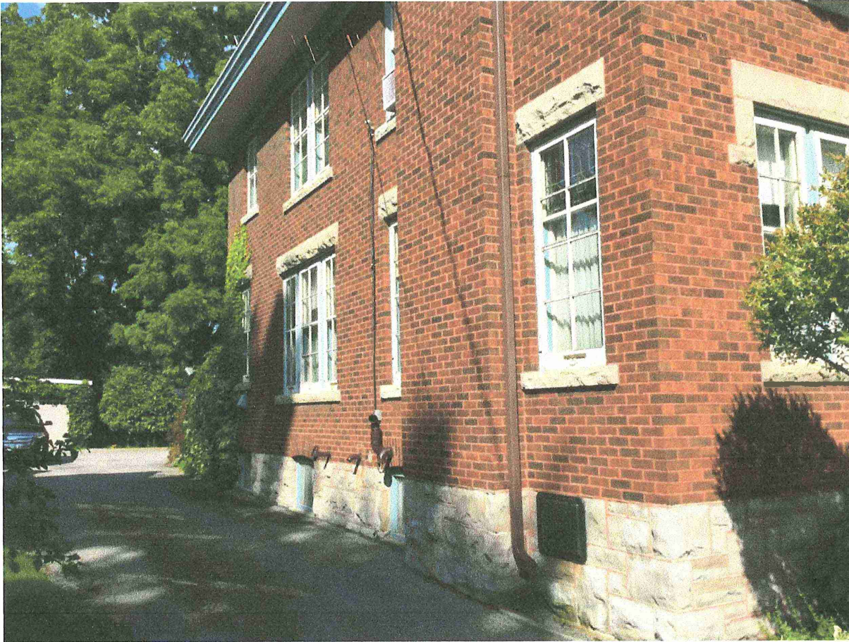
VIEW OF FRONT OF HOUSE AND DRIVEWAY SIDE SHOWING 'FOUNDATION' STONEWORK AND WINDOW DECORATIVE STONEWORK - TYPICAL FOR ALL HOUSE WINDOWS – WITH THE EXCEPTION OF THE STACKED SUNROOMS (EAST SIDE)
