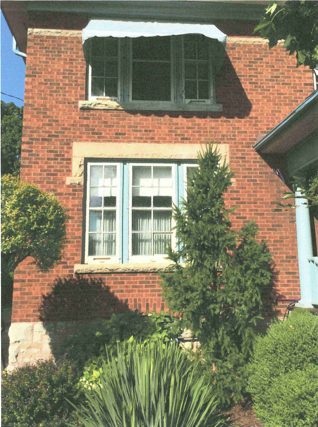
STONWORK ABOVE AND BELOW MAIN LIVING ROOM WINDOWS
