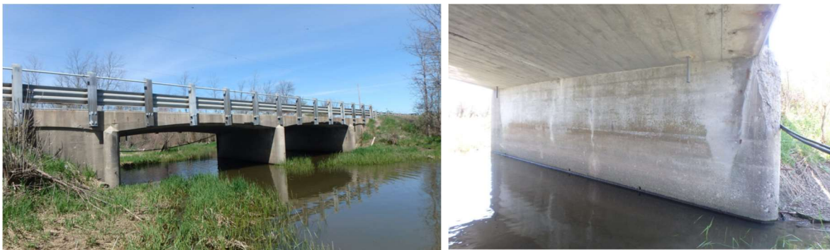
Figure 28 Lakeshore Road Culvert (BCI=93 Very Good)
