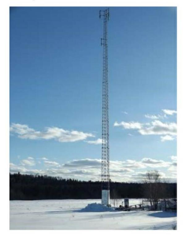
The tower will be a 45m lite duty self support lattice tower. It will have a footprint of 3m x 3m. There will not be a building at the base of the tower.
