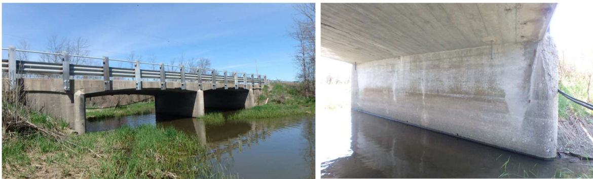
Figure 28 Lakeshore Road Culvert (BCI=93 Very Good)
